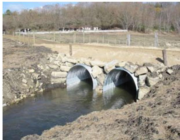
Note the change in water height within the culverts which allows for fish migration.
