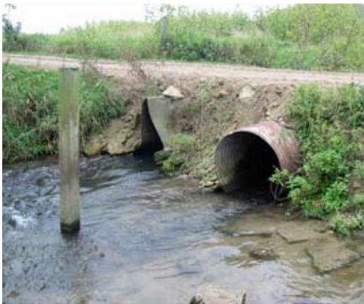
Perched culverts before installation of replacement culverts.
