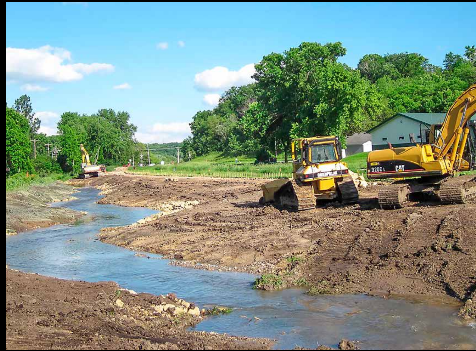
Creating the new stream channel 2013.
